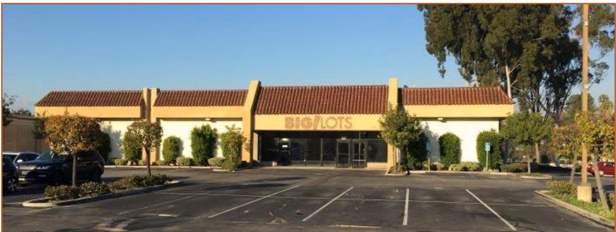
Note: Opportunities for new user(s) in former Big Lots building.
